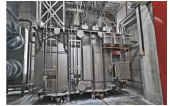
A 50 MVA power transformer outfitted with compact Connex connections in an underground transformer cell of the new Oerlikon substation.
