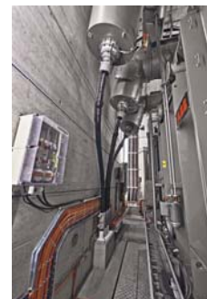
Safe to the touch, even when high voltage is applied: Three cable connections to the 50 MVA transformer realized with the encapsulated HV Connex system for 170 kV applications.
