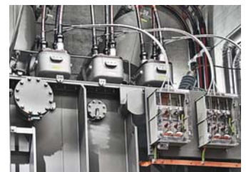
Ultra compact: Several vertically routed medium-voltage cables can be connected to the new Connex transformer terminals rated to 52 kV.
