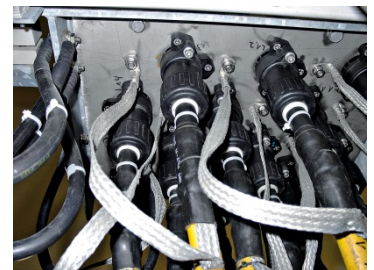
PLUG allows the simple pre-assembly of tower cabling in wind energy plants.
